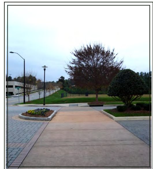
Example of a Pedestrian Refuge Island in Raleigh, NC
